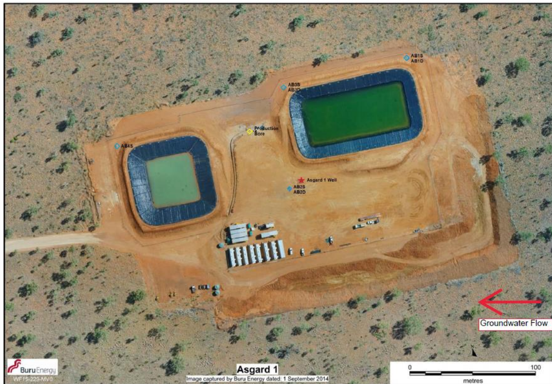
Figure 5-28: Location of VNB4S / VNB4D and AB1D / AB1S and proximity to existing infrastructure
