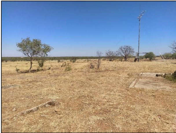
Figure 5-50: Legacy pastoral station buildings with radio tower (can be seen from Calwynyardah–Noonkanbah Road ~700 m away)
