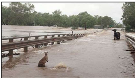
Figure 5: Fitzroy Crossing Bridge during the flood 1
