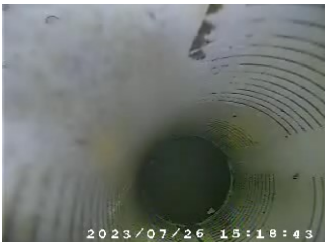
VNB4S bottom of well of 42.3 m btoc.
