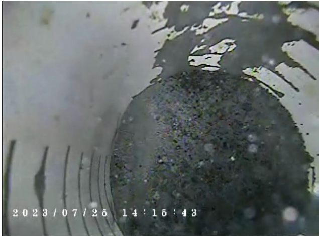
AB1D debris build up on casing wall and bottom of well.
