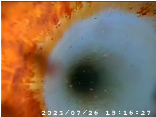
VNB4S casing below SWL of 30.686 m btoc.
