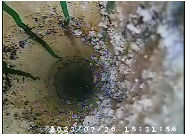
VNB4D debris below SWL at 30.956 m btoc.
